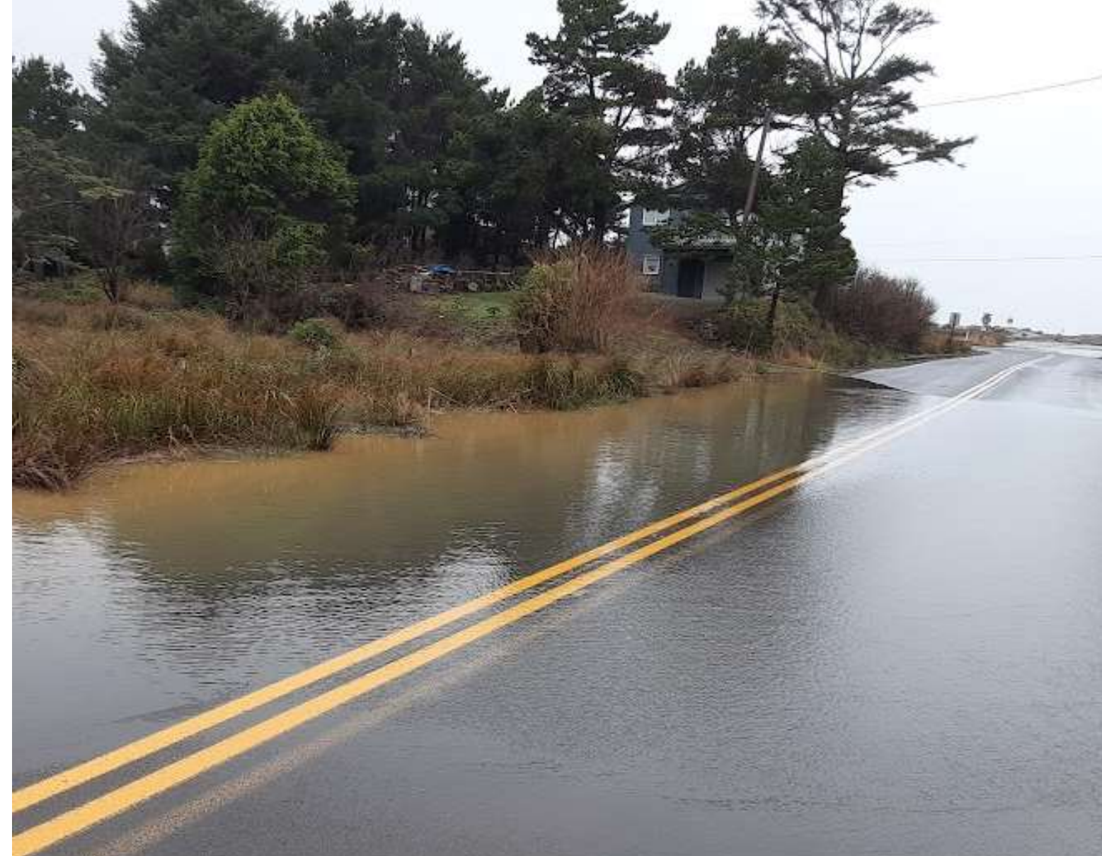
By design, floodwater flows over the road at concrete spillway
