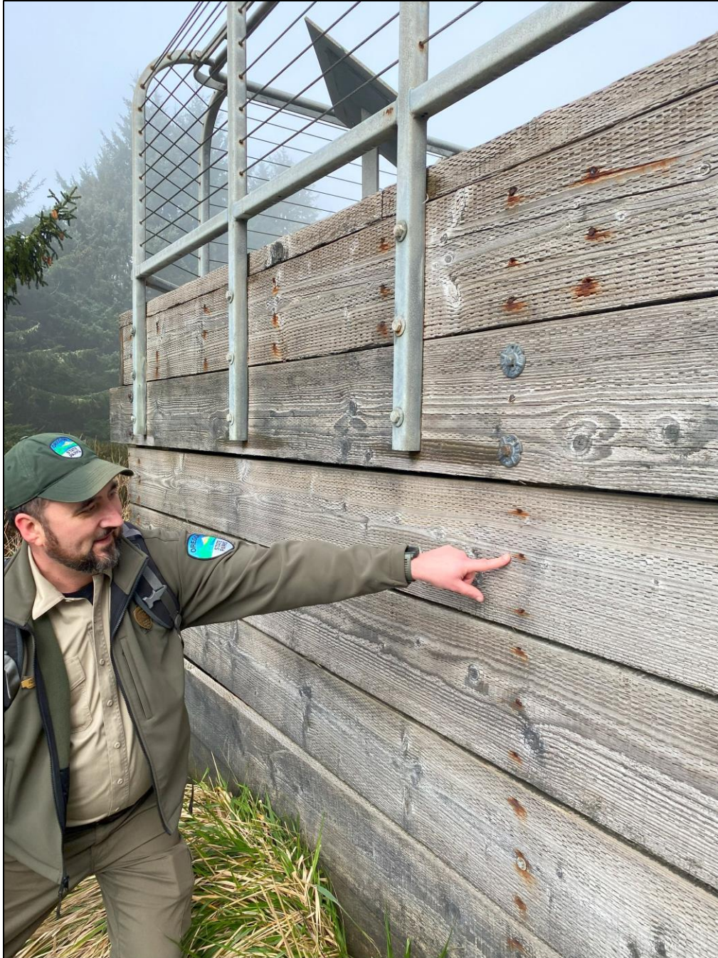
Figure 35. South overlook area showing degraded wood and nails.
