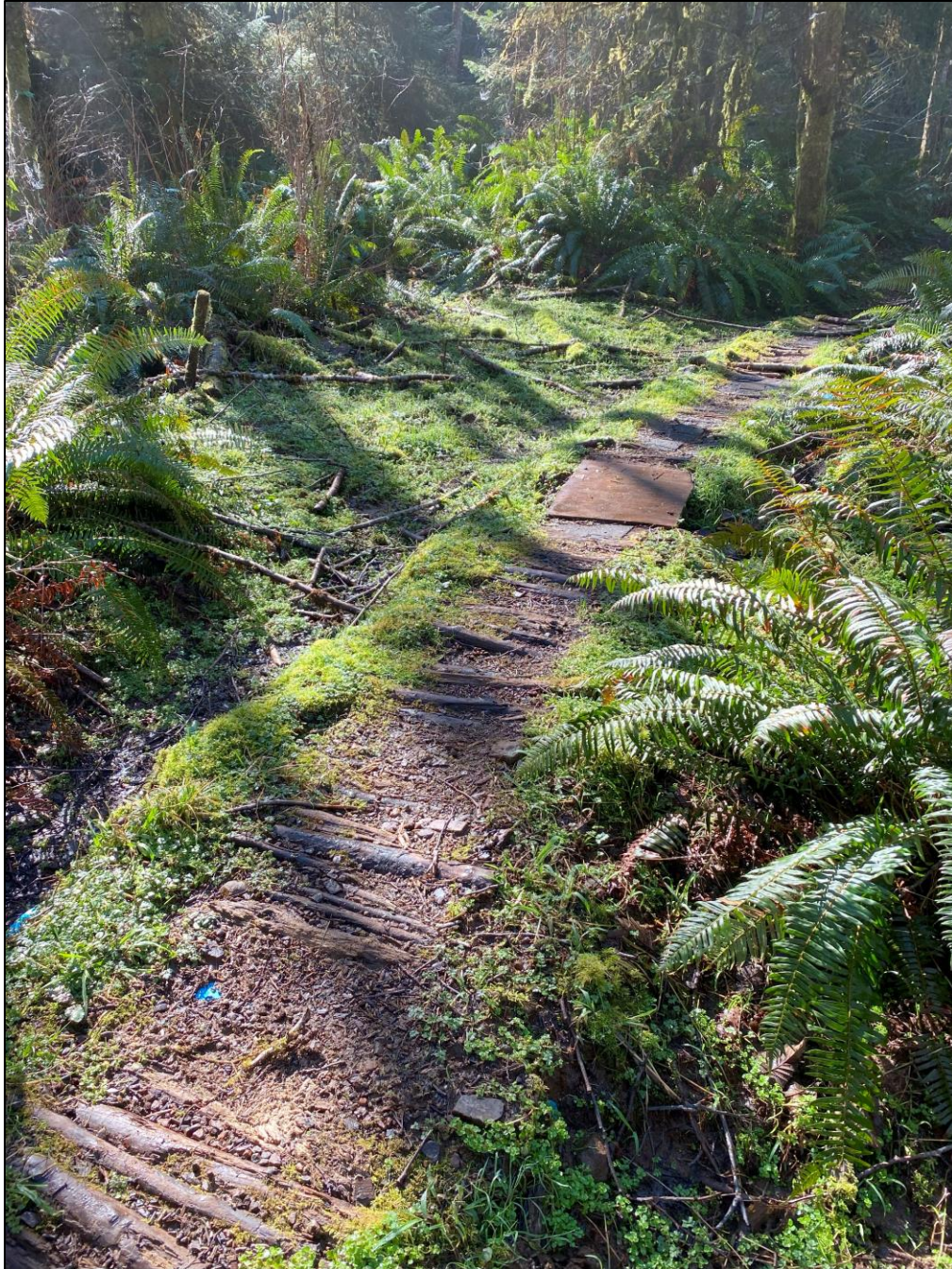
Figure 23. User-created corduroy trail on Nascowitzen trail.
